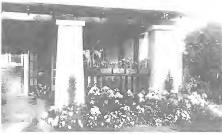
Coolibah, Hunters Hill, showing use of window boxes to soften a verandah.
